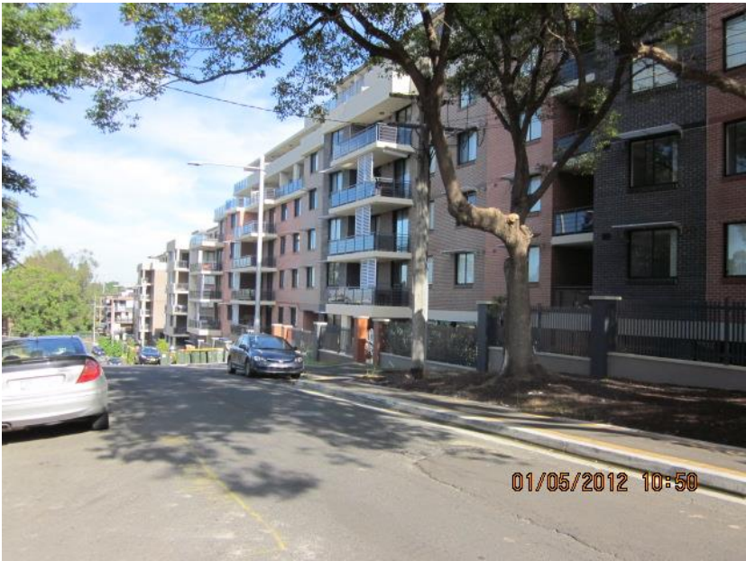
Photograph 1: The photograph demonstrates the existing buildings opposite in 82-84 Porter Street (Bay One Development). The buildings range in height from seven storeys down to five storeys towards the foreshore.
