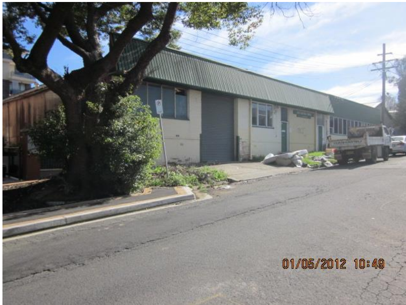
Photograph 3: 2-4 Porter Street. A recent approval has been granted for a two x six storey mixed use development.
